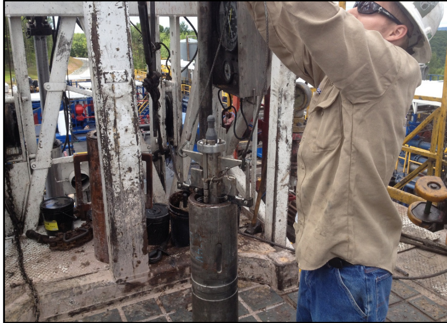
Figure 25 Pickup sling on the Gap sub box
