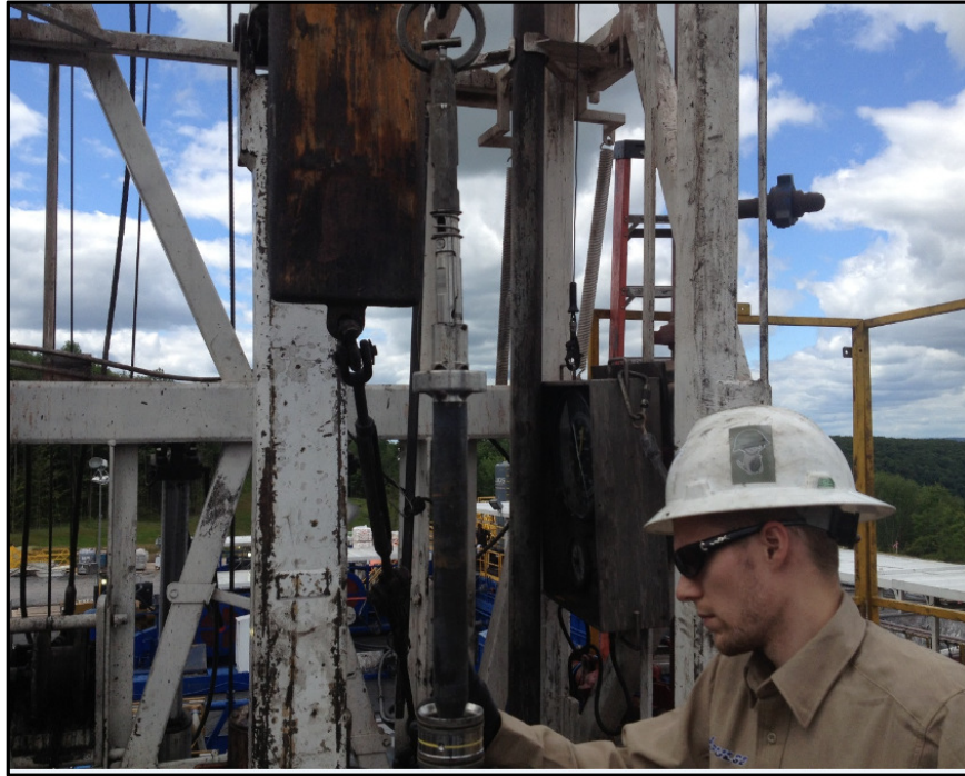
Figure 28 Pickup the DPG above the collar
