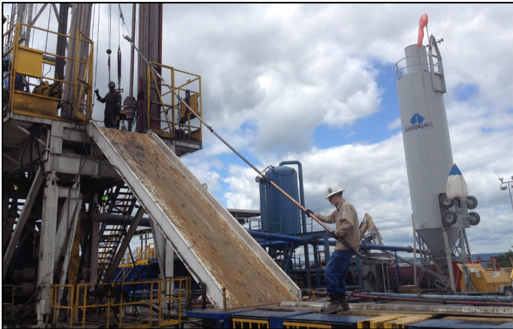
Figure 20 Walk the Tool up the V-Door
